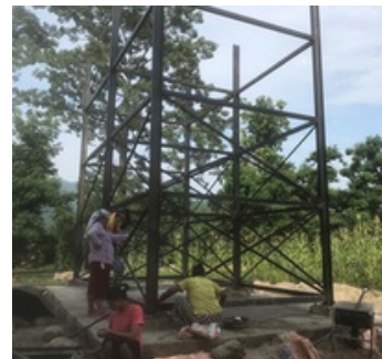
Tower Frame Assembly
