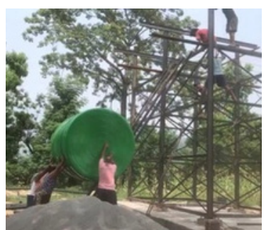
Tank Installation
